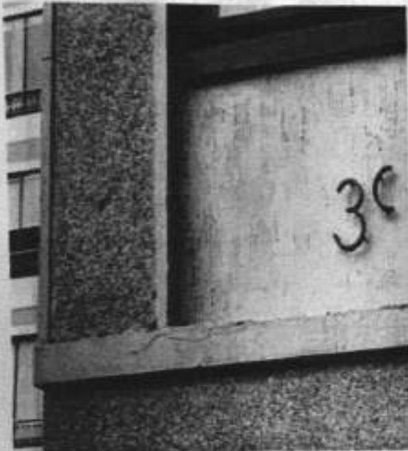
**FIG. 2 FISURA EN FACHADA**
