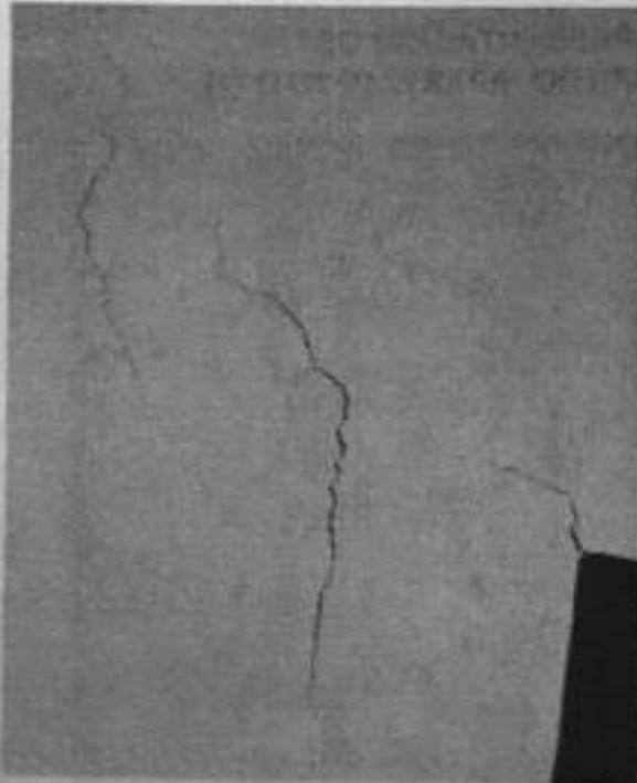
**FIG. 36 FISURAS PARTE
