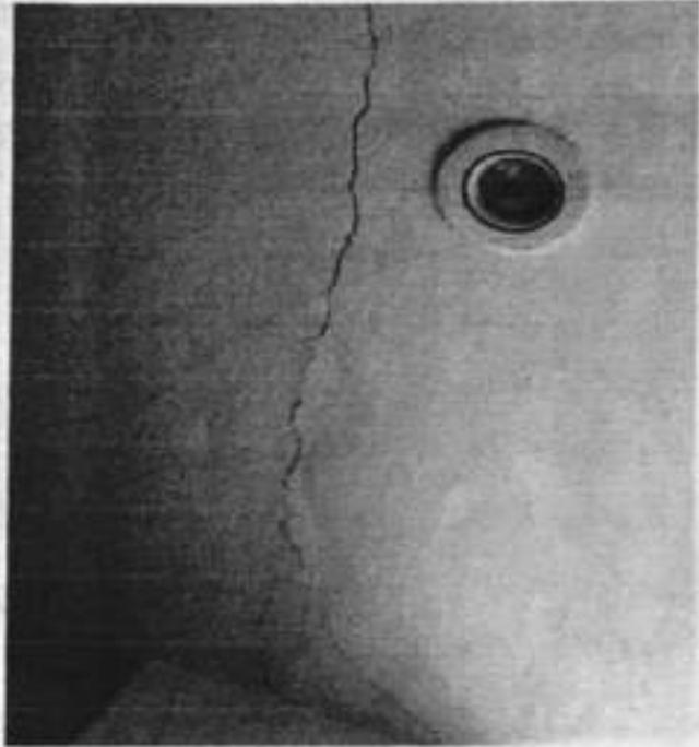
FIG. 39 FISURA TECHO APTO. (2)
