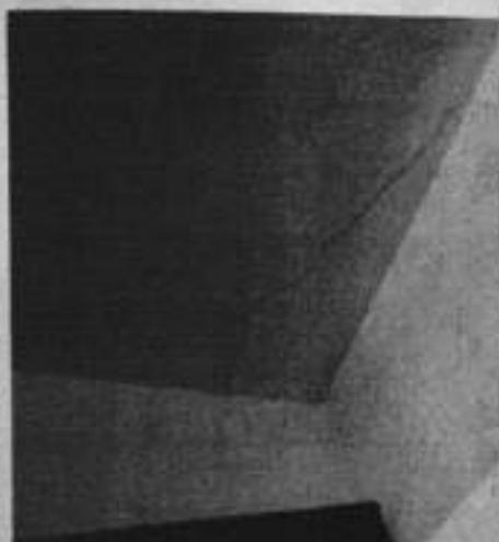
FIG. 20 FISURA EN TECHO
