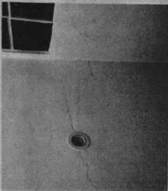
FIG. 53 FISURA TECHO APTO. (2)
