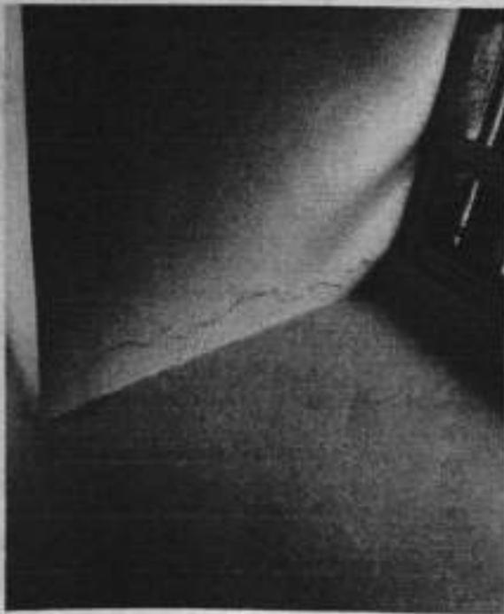
FIG. 51 FISURA TECHO APTO. (2)
