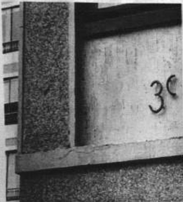
**FIG. 2 FISURA EN FACHADA**
