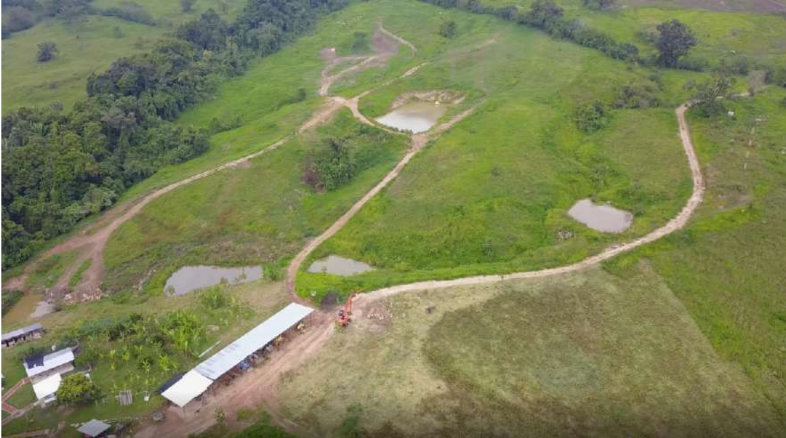
Reservoirs, machinery workshop and warehouses Reservorios, taller de maquinaria y bodega
