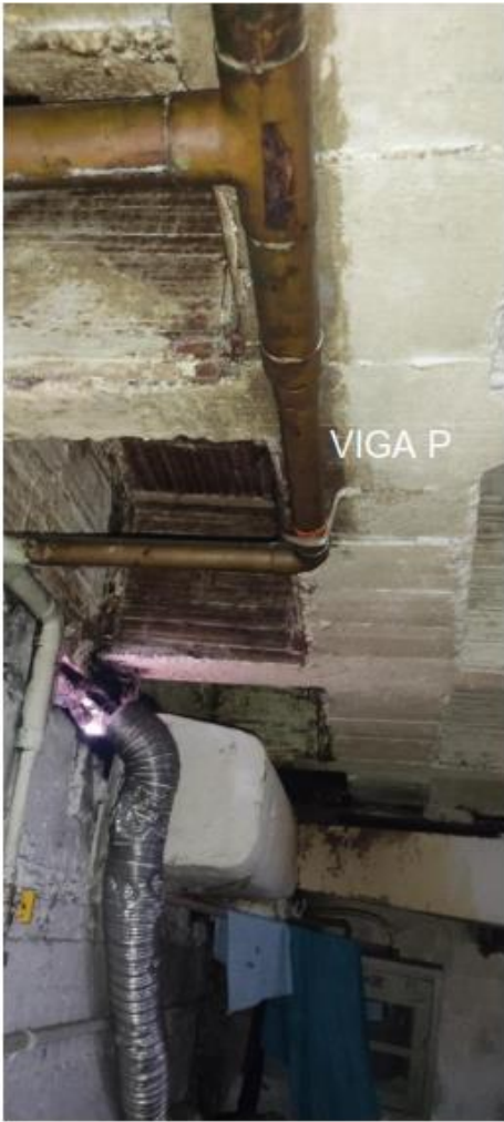
VIGA PORTICO PRINCIPAL
