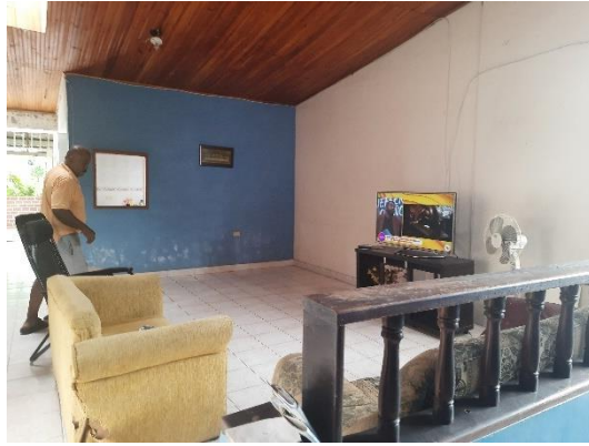
Detalle sala principal piso 2
