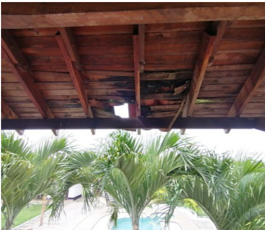
CIELO RASO CASA PRINCIPAL PISO 2
