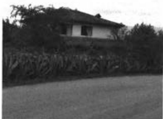
VISTA FRONTAL EXTERIOR
